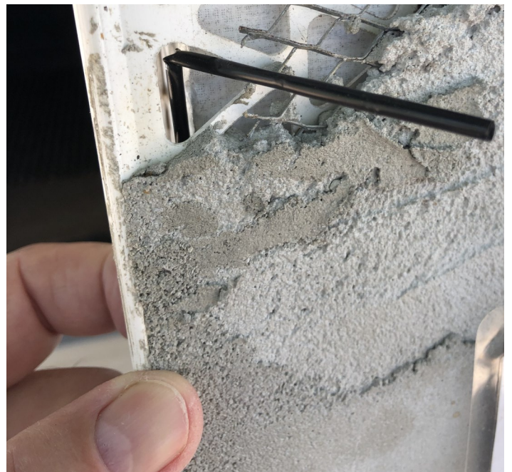
Figure 8-3 - Coffee stirrer shown above slid down into the cavity created by Vinyl Corner Bead's Nosing/Flange Intersection area
