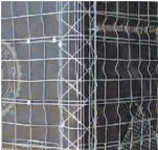
Figure 8-5 Preformed Wire Reinforcement
