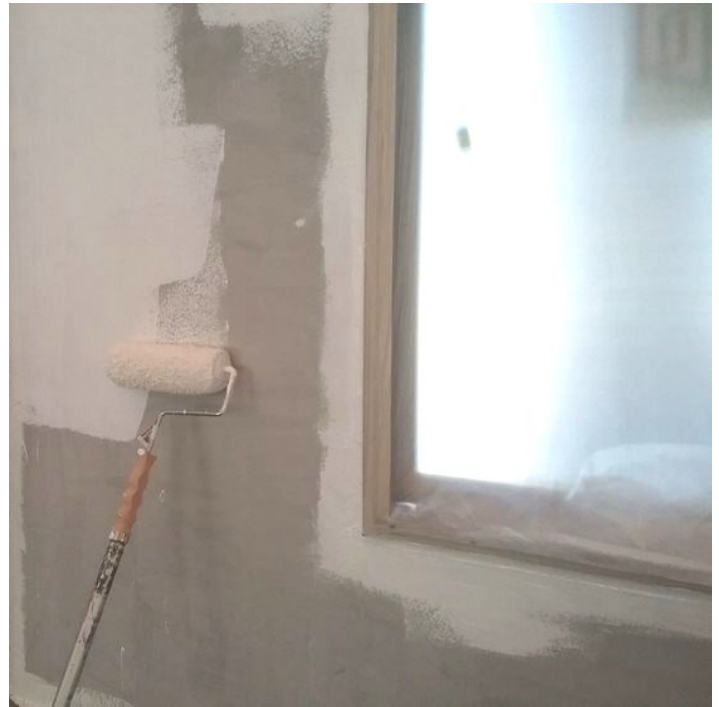
Figure 10-5 Apply 2nd Coat of Drylok Extreme. Roll or Spray according to the application processes and thickness as described in previous chapters
