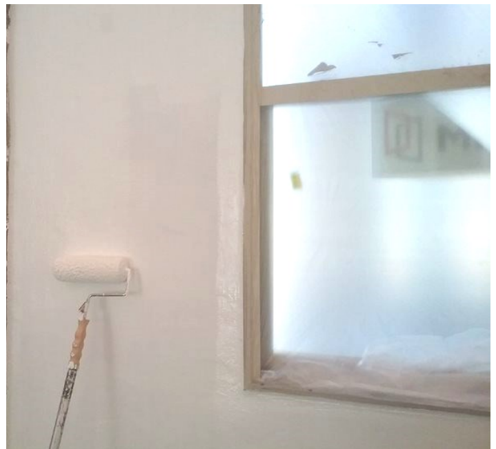
Figure 10-5 Apply 2nd Coat of Drylok Extreme. Roll or Spray according to the application processes and thickness as described in previous chapters
