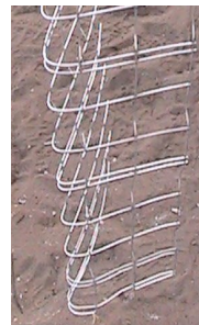
Figure 8-27 StructaLath Jobsite Made Preformed Outside or Inside Corner
