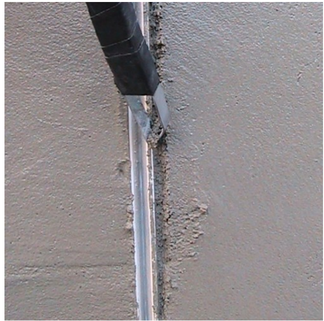
Figure 7-5 Cutting the Sealant Socket with the "V" tool. Two (2) - 3/16" deep passes are made to ensure a smooth socket
