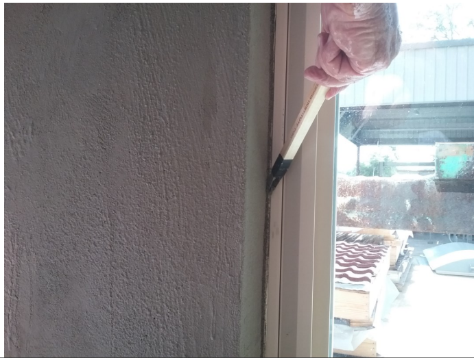
Figure 8-18 "V" Tooling a sealant seat at a masonry window return
