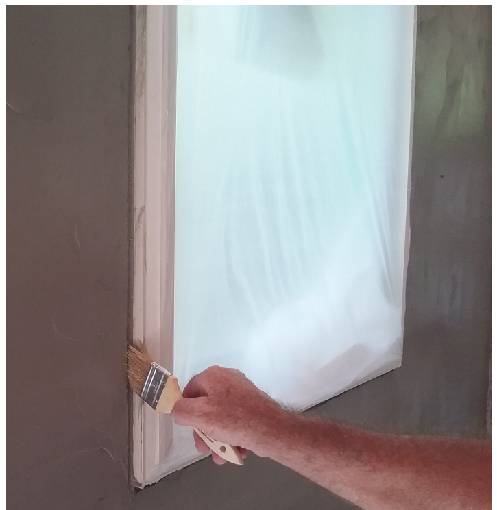
Figure 8-21 Brushing the "V" socket to smooth edges, clean shoulders and seal for application of tooled sealant on frame wall with fin window
