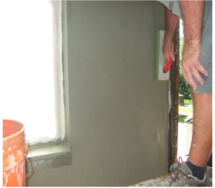
Figure 8-17 Using a soft closed cell float (slide up and down) to gently form a slightly rounded corner.
