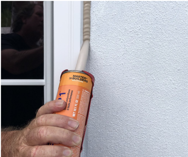
Figure 7-10 Application of Approved Sealant
