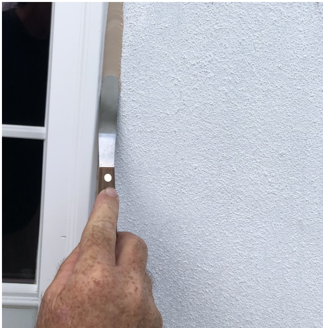
Figure 7-12 Spatula presses sealant into socket forming a sealed bond and smoothing the face for final coating applications
