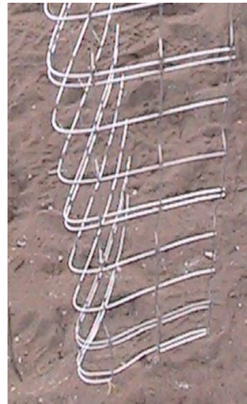
Figure 8-7 StructaLath Wire Bent Around Corner as a Continuous Application
