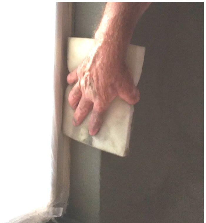
Figure 8-17 Using a soft closed cell float (slide up and down) to gently form a slightly rounded corner.
