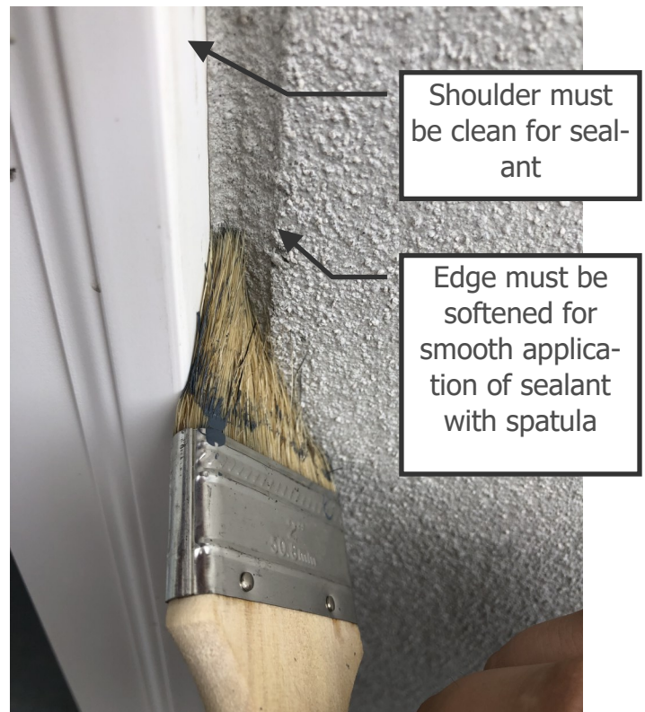
Figure 7-9 Brush bristles are angled to smooth the socket seat, smooth over the top edge and clean the shoulder of the penetration
