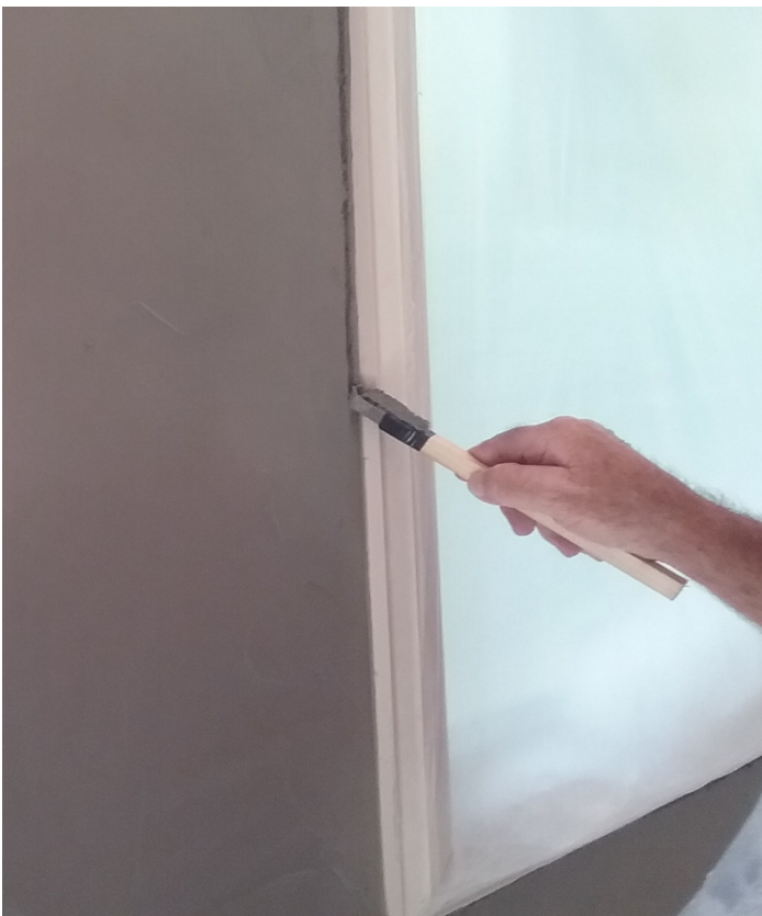
Figure 8-19 "V" Tooling a sealant seat along the shoulder of a fin window in frame wall
