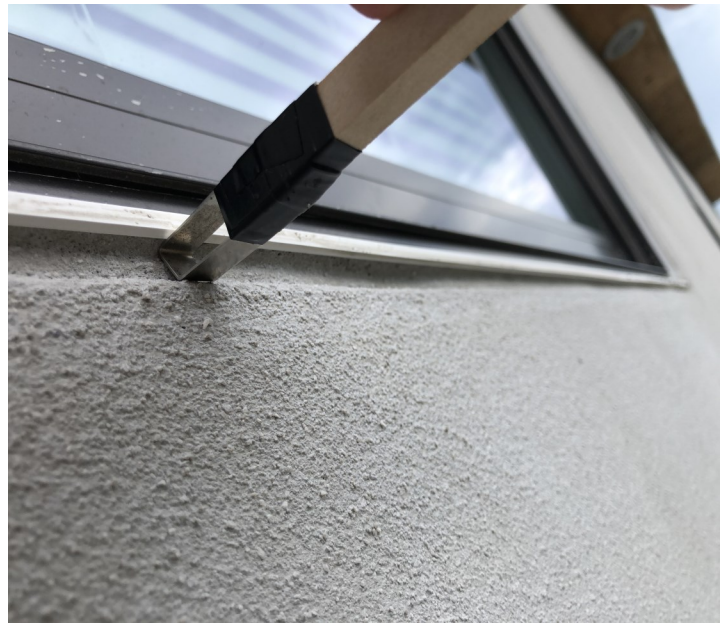
Figure 7-9 Brush bristles are angled to smooth the socket seat, smooth over the top edge and clean the shoulder of the penetration
