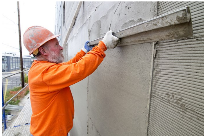
Figure 9-2 Setting "Dots" to a line for Dot-and-Screed straightening. Alternate to control joint screeding.
