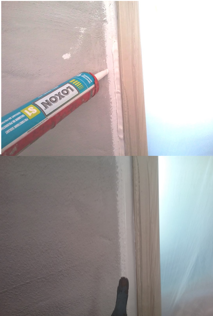
Figure 10-3 After priming socket seat, apply Sealant and Tool with Spatula
