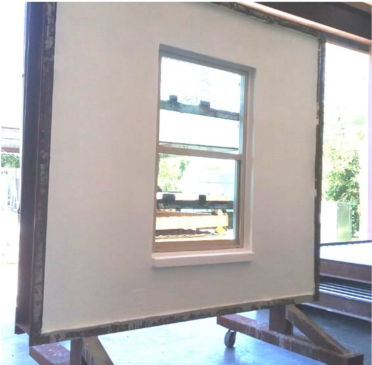
Figure 10-6 One of the walls finished and ready for full scale testing and modeling.
